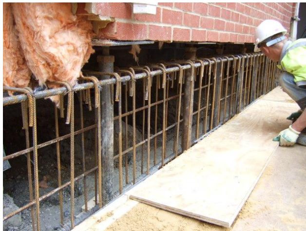
Fig 3: Beam Reinforcement
