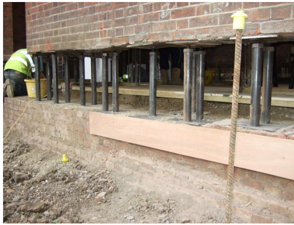
Fig 16: Installation of a ground beam using stools
