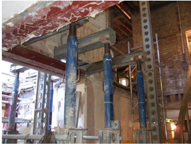
Fig 14. Temporary works - support to existing structure
