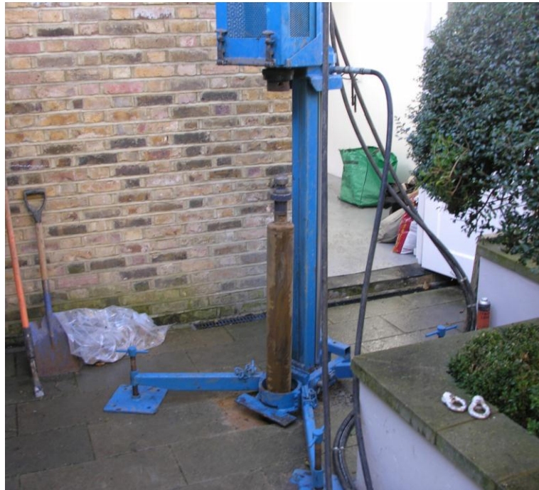
Fig 27: Restricted access modular site investigation rig
