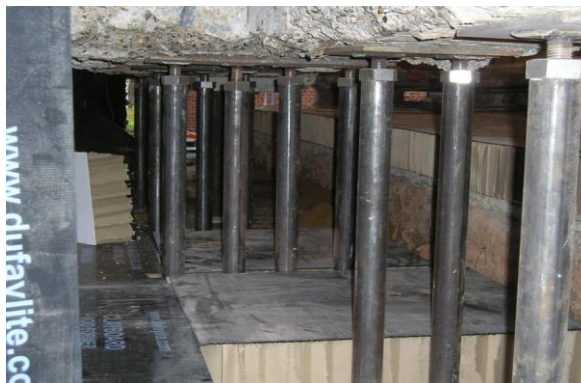
Fig 18: Installation of adjustable stools or props
