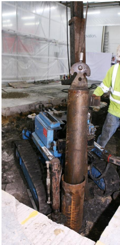
Fig 22: Driven pile using a drop hammer rig
