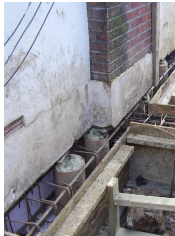
Fig 9: Piles to support vertical loads
