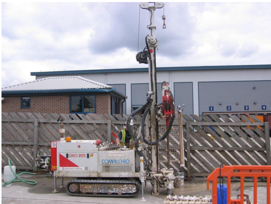
Fig 28: Full access site investigation drilling rig
