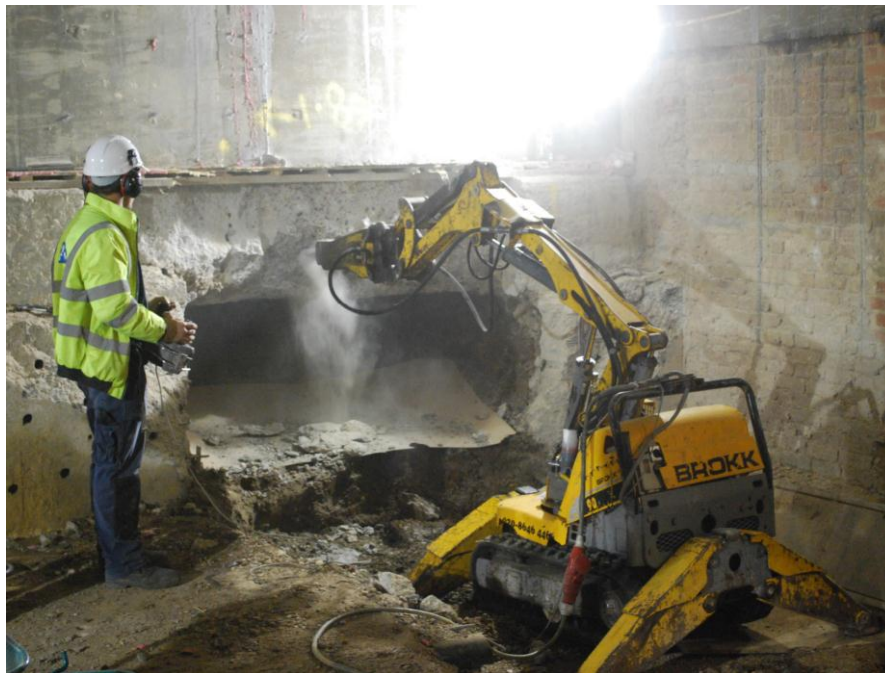
Fig 24: Concrete break out
