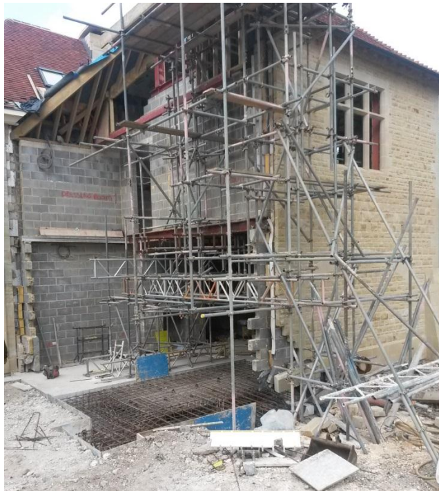
Fig 15: Temporary works - support to existing structure
