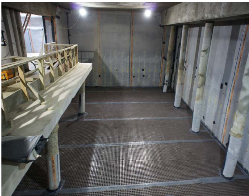
Figure 47. Cavity membrane after installation in a basement
