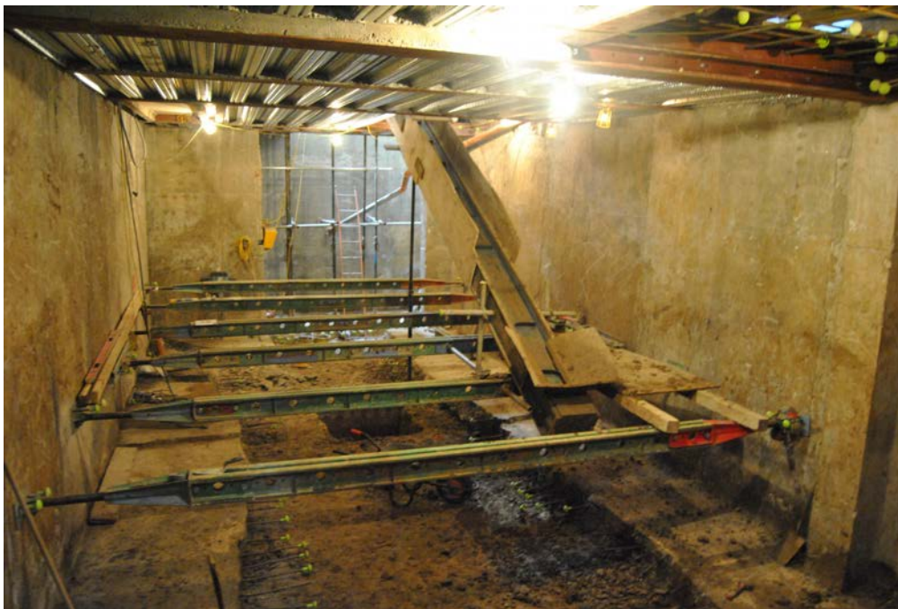
Figure 30. Temporary works - main excavation
