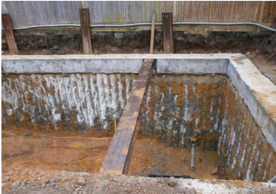
Figure 20. Secant piled wall
