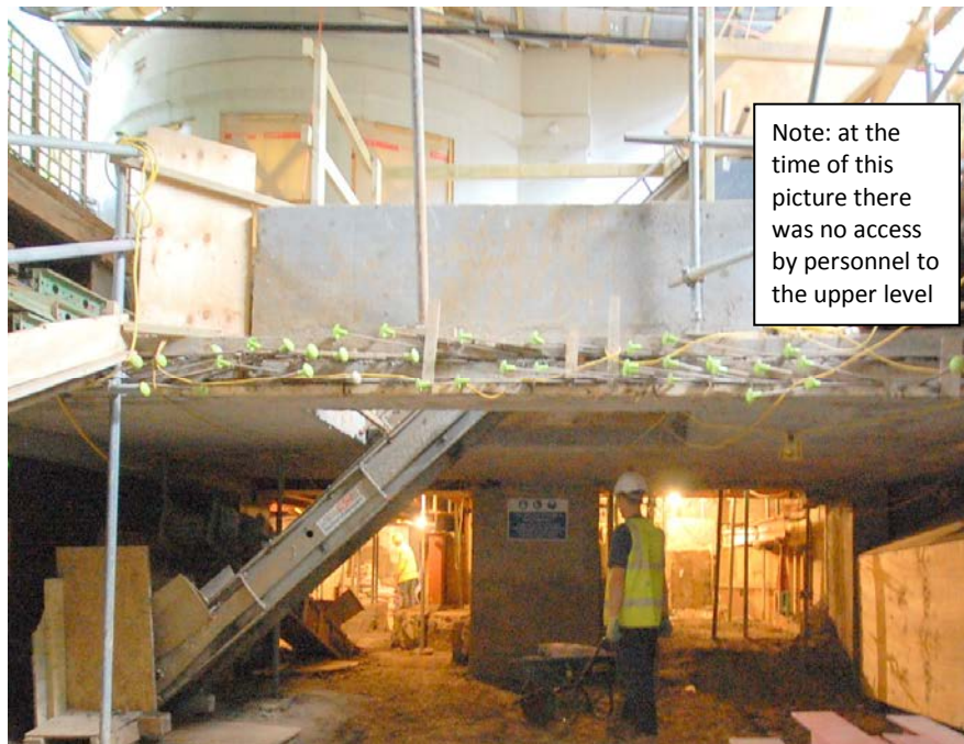
Figure 37. Tunnelling under occupied house
