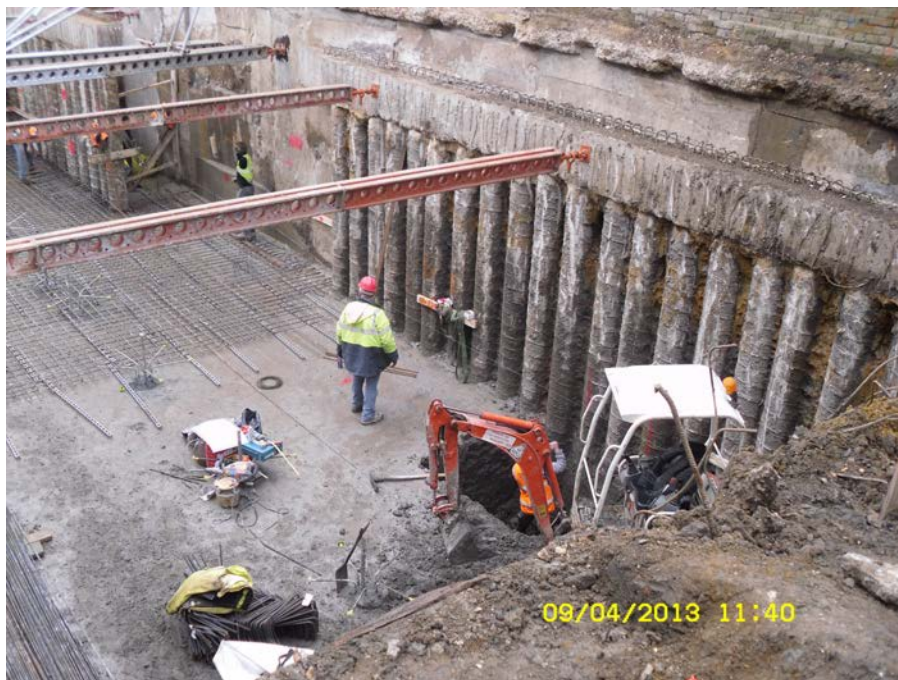
Figure 18. Contiguous bored pile wall
