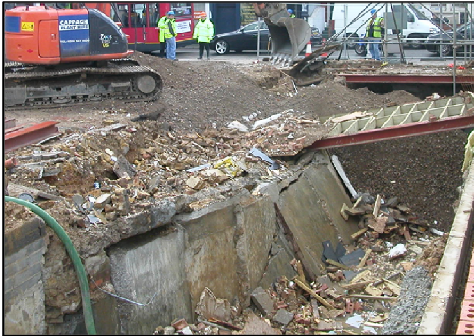
Figure 7. Wandsworth, South London during construction of a basement - effect of horizontal force from the ground on unrestrained basement wall
