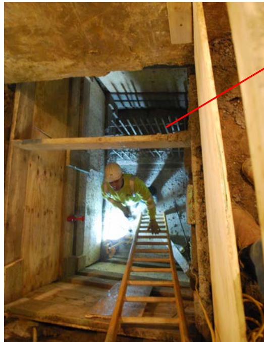
Figure 6. Underpinning - Access shaft used to construct a single underpin – note the small work area and the temptation to limit the amount of shoring materials. The foot of the pin has been cast and steel reinforcement for the pin is being installed. Contrast the less than ideal support arrangement with the standards shown in Fig 28 on page 37.
